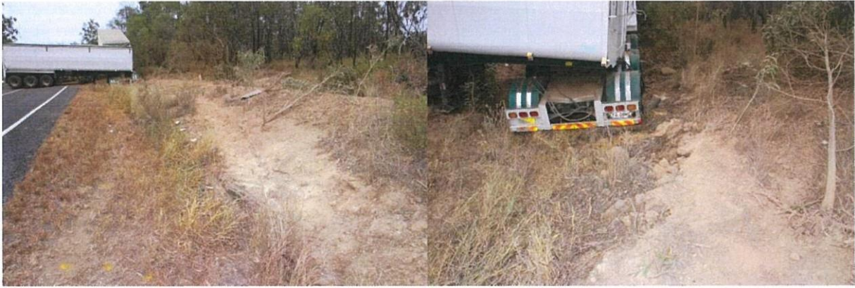
Image showing the western edge roadside drainage and wheel marks through vegetation with tree damage leading to drainage ditch roadside bottom of decline western side.
