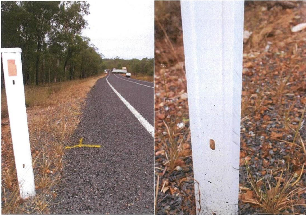
Scuff indicating first observed point of contact on roadside reflector post.
